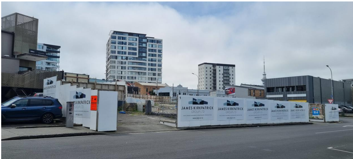
Figure 4 - looking north towards the main 538 Karangahape Road site from Abbey Street
