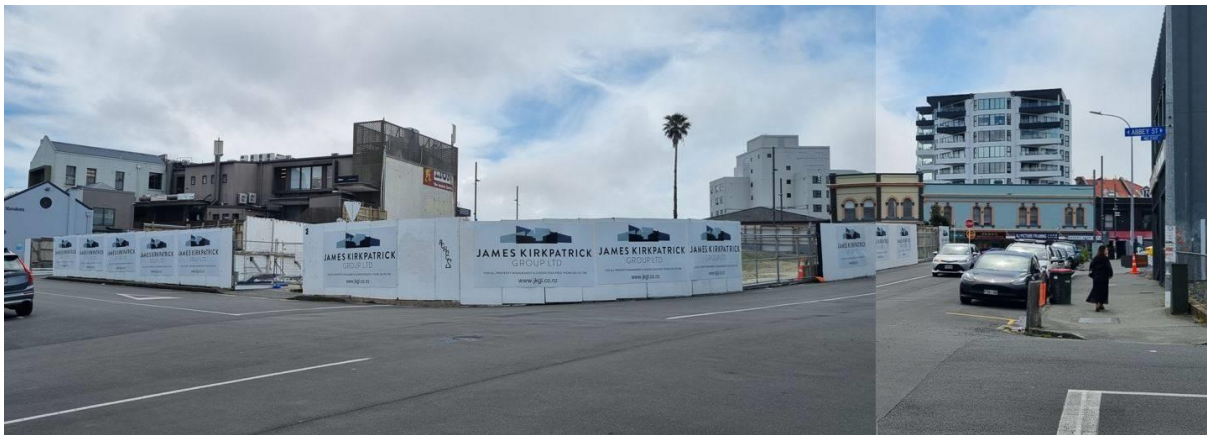
Figure 5 - Looking north-west across the site from corner of Abbey and Gundry.
